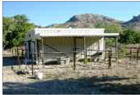
Covered pens surround the combined shower, laundry and hay barn at Hilltop Hideaway.
